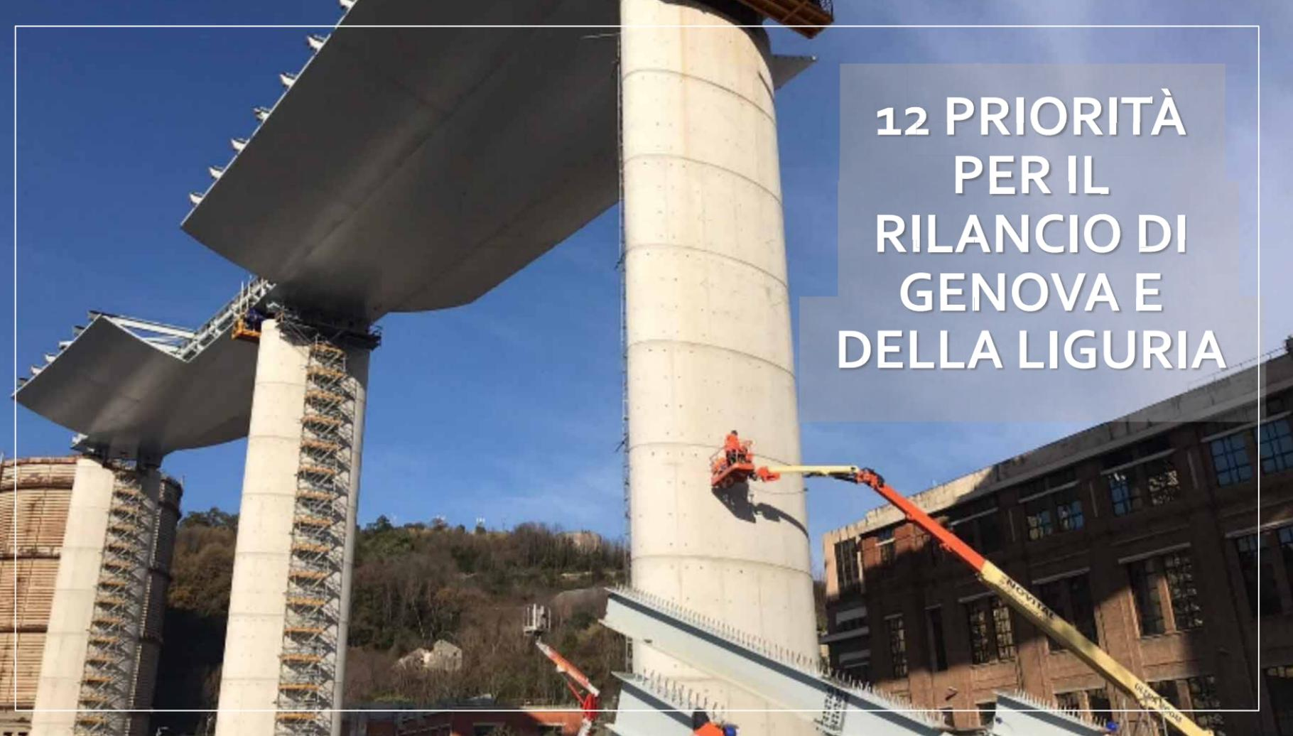
A photograph of a bridge under construction. The image shows several large, cylindrical concrete pillars supporting a wide, flat bridge deck. Scaffolding is visible around the pillars, and a worker in an orange safety vest is on a yellow crane bucket positioned against one of the pillars. In the background, there is a multi-story brick building and a hillside with trees. The sky is clear and blue.
